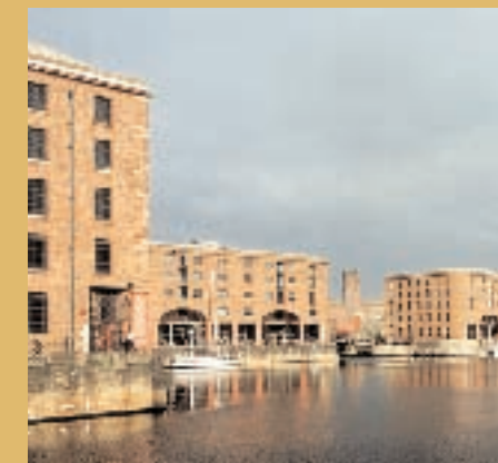
6. Albert Dock Warehouses Opened 1846/7 Grade I Opened 1846-47 Albert Dock Warehouses form the largest group of Grade I Listed Buildings in England. Jesse Hartley used well-established techniques adapted from textile mill methods. He introduced new solutions, such as the amazing stressed-skin iron roof. Raising of goods from the quaysides was performed with the first hydraulic cargo-handling installation in the world.
