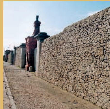
10. The Dock Wall Its purpose was to control rather than prevent access from the town into the docks, and the monumental gateways with their heavy wooden gates sliding in iron guide rails effectively made the docks into a fortress-like stronghold. The design of the various gate piers demonstrates a fascinating progression from Foster's early classical style to Hartley's whimsical turrets.
