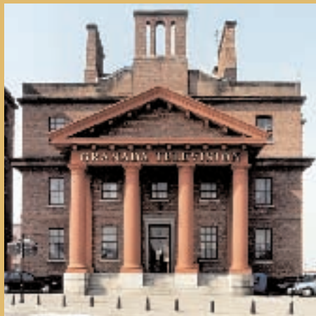
7. Albert Dock Traffic Office 1846-7 Grade I This is one of a number of building designs by Hartley in collaboration with Philip Hardwick. It is built of brick with red sandstone dressings. The most remarkable feature is the cast iron Tuscan portico and frieze. The building was restored by the Merseyside Development Corporation and re-opened as television studios.
