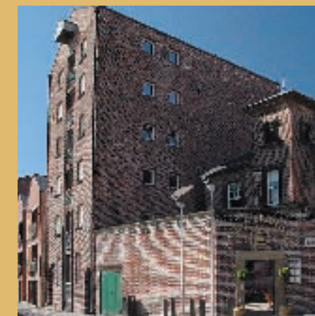
19. The Bridewell 1861 Grade II Located in the Duke Street area, the Bridewell, or Police Station, dates from c.1850. It is of brick with stone dressings and a slate roof. The building is of two storeys and three bays, with the centre bay projecting to form the base of a short tower. The Bridewell is now a public house and restaurant.
