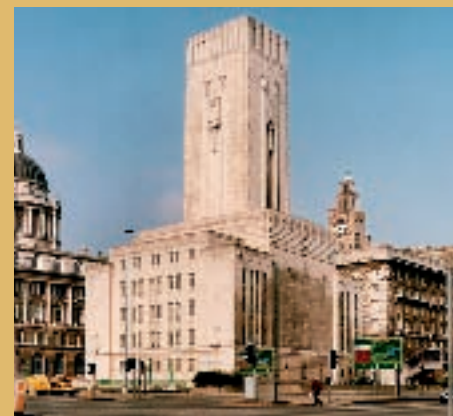
4. George's Dock Tunnel Ventilation Building and Offices 1931-1934 Grade II This stylized obelisk, reminiscent of ancient Egypt, was designed by Sir Basil Mott and J. A. Brodie, with Herbert J. Rowse, to serve the Mersey Road Tunnel. It has statues of Night and Day, symbols of the never-closing Mersey Tunnel and a black marble memorial to the workers who died in its construction.
