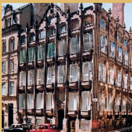
14. Oriol Chambers 1864 Grade I Designed by Peter Ellis, the use of oriel windows was driven by a desire to provide good daylight. The oriels themselves are framed in the thinnest sections of iron. In its day, the building aroused much opposition. It is only recently that its futuristic qualities have become appreciated.
